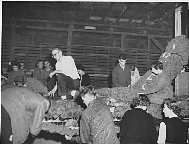
Prepared under shelter . . .
