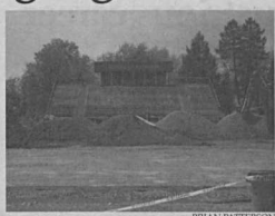
The field in Scott S. Bair stadium is undergoing a transformation from natural grass to synthetic turf. Large piles of gravel are being laid as a base for the turf.
