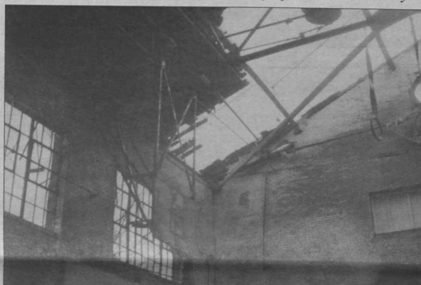
The fire consumed most of the roof, as seen here, and hollowed out the building, leaving only an empty shell. Contracted disaster cleanup will be taking place over the next few weeks and a new roof will be constructed.
