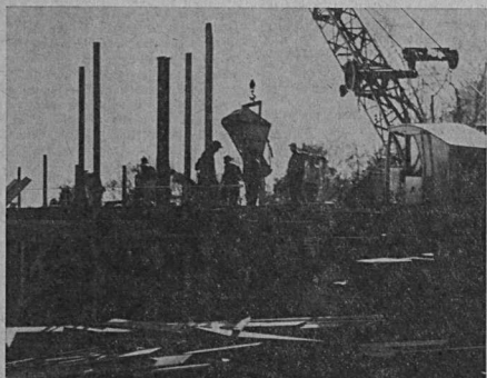
THE HUGE STEEL boom of the derrick slowly lowers the cement bucket into place.
