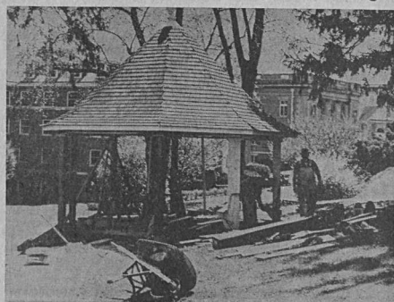
CARPE DIEM GETS A NEW LOOK as workmen renovate the octagonal portico between McDaniel and Science Hall. The supporting, initial-covered posts which long have threatened to tumble have been replaced with sturdy new ones. New benches will be installed and the structure will be brightened with paint.
