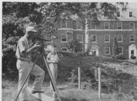
Sighting the line following excavation.
